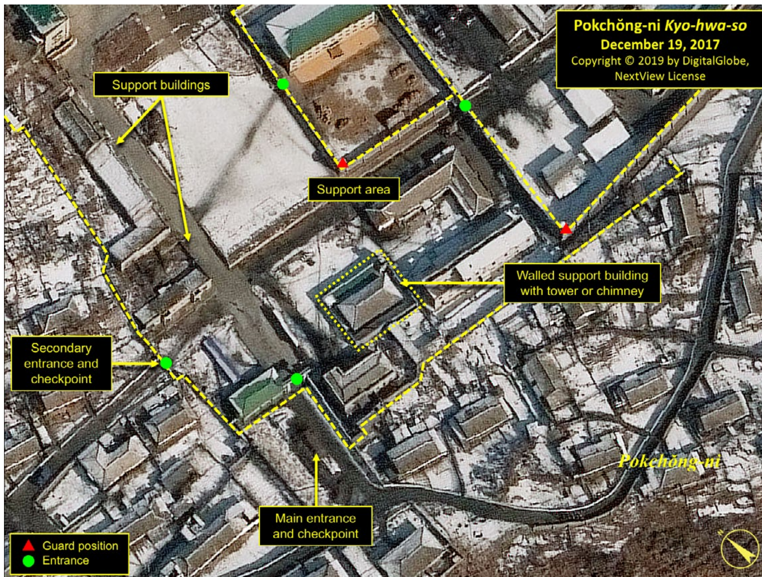
A close-up view of the support area on the south side of the facility on December 19, 2017. Of note is a small building surrounded by a high wall and a small elevated structure (potentially a guard tower or chimney) attached to it.
