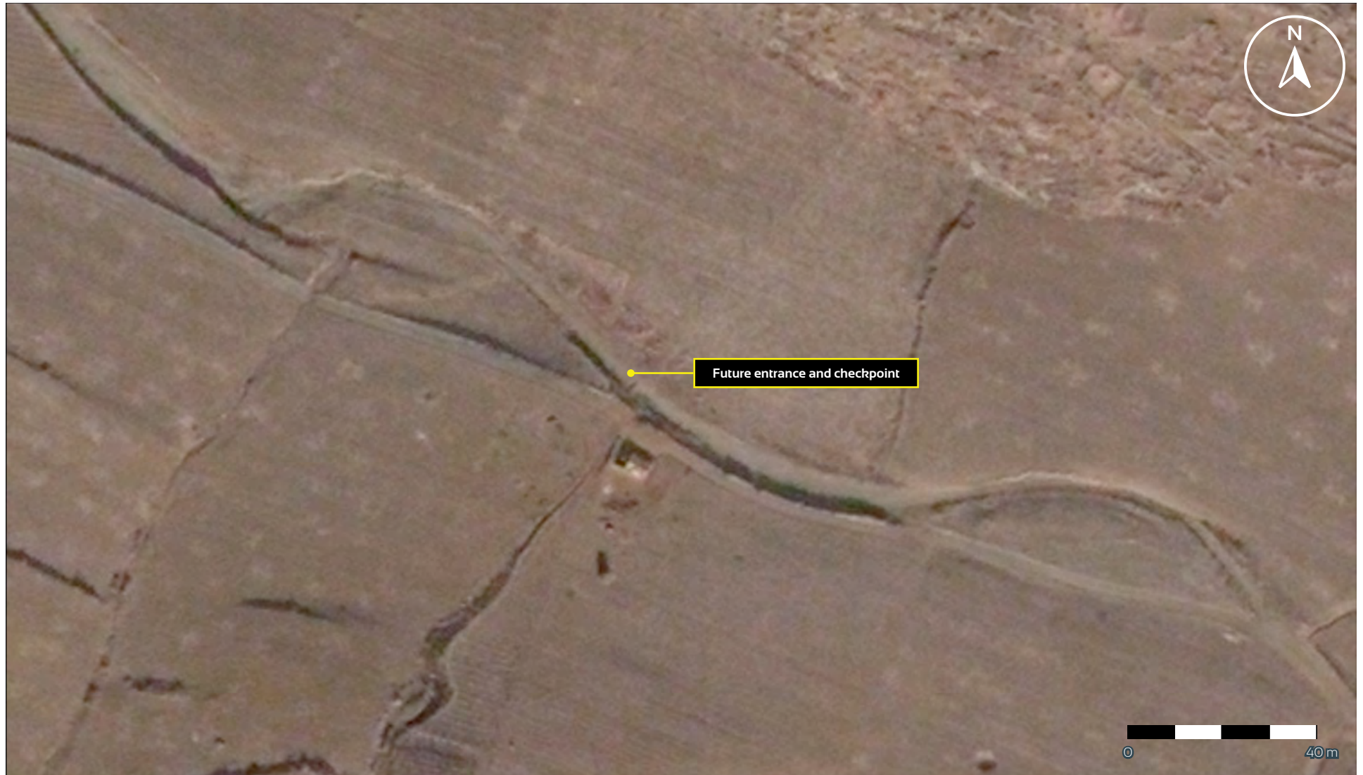
Area 10 - Secondary Facility Entrance and Checkpoint West (125.961293, 39.646120)
